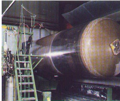
1 Manufacturing of an underground petrol storage tank Application of the corrosion resistant liner resin
