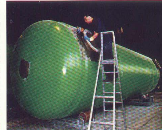
4 Laminating the manhole
